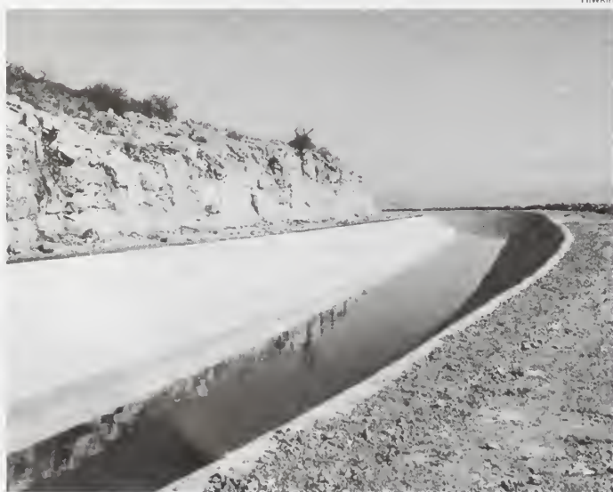
Figure 4: One of the modern concrete-lined canals of the Israel National Water Carrier that carries water from Lake Tiberias in the north to the Negev, the arid lands of the south.
